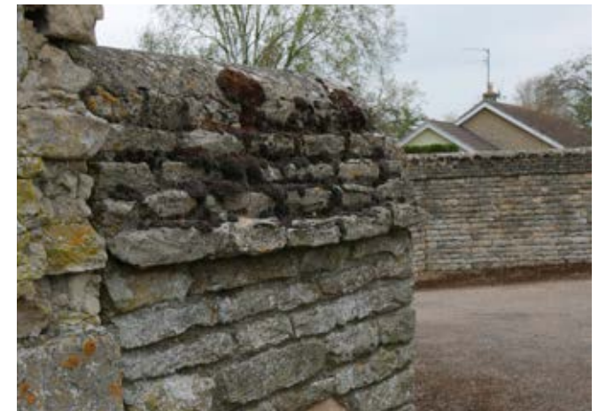
Close up of limestone masonry wall on Church Lane
