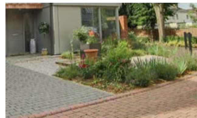
Permeable block paving in different colours and planting to define spaces for parking
