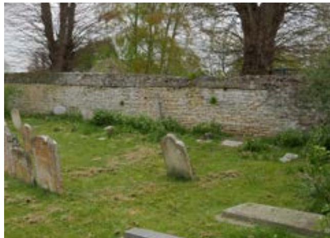
The church wall in limestone masonry with Collyweston tile parapet
