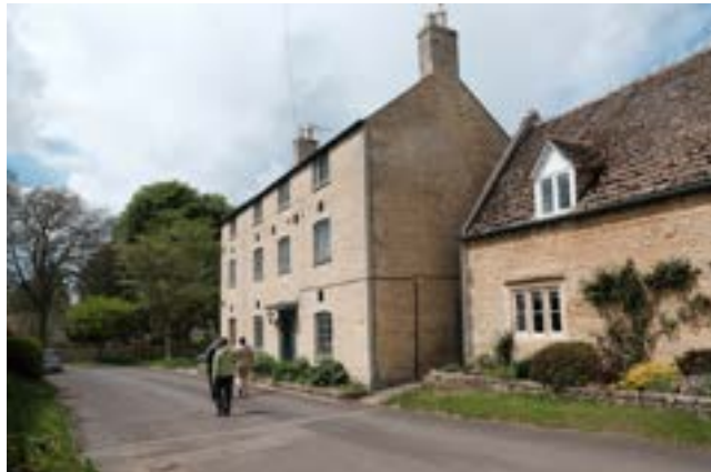
The three storey old Laundry building
