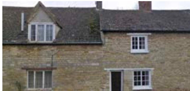
Timber white casement windows with exposed lintels, three-sash dormer
