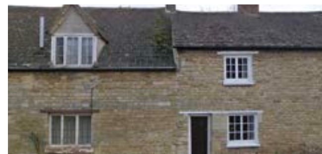
Timber white casement windows with exposed lintels
