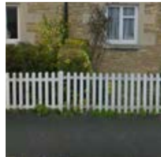
Low timber picket fencing
