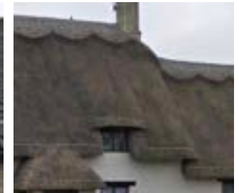
Thatched roof and small dormer
