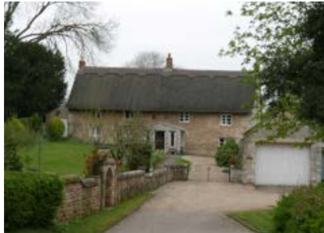
The Spinney, a C17 farmhouse made of rubble limestone and dressed stone corners with thatched roof.
