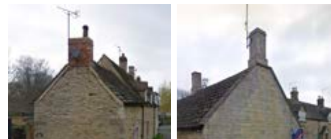
Red brick and stone chimneys located at the ends of prominent gables
