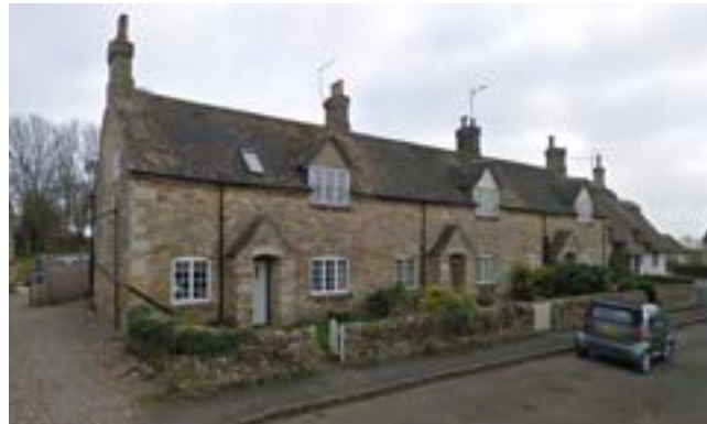
Gable end chimneys, protruding porches, prominent wall dormers and stone garden wrapping wall
