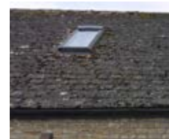
Collyweston tile roof and skylight
