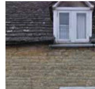
Typical stone building and casement dormer
