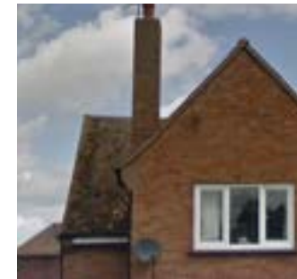
Exposed red brick building
