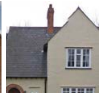
Rendered brick building
