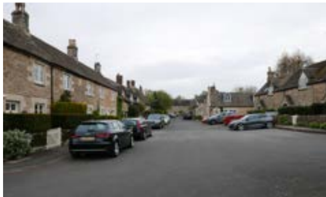
Well Cross terraces
